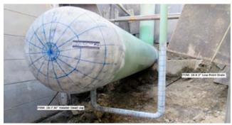
An example of a header deadleg and low point drain excavated for inspection. [3]
