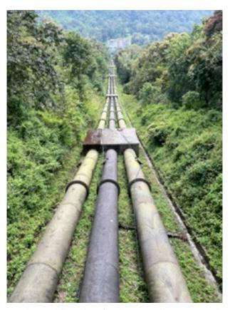
Figure: Above-ground oil/gas pipeline in a forested area. Remote pipelines may require periodic III pigging for data-rich assessment, or alternately ECDA surveys if shutdown or pigging is impractical. ECDA is a "continuous improvement process" and part of the asset management plan for such pipelines
